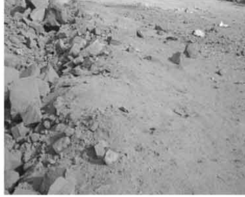
5 Pre-splitting blast without back-break behind pre-splitting row, test no. 2.
